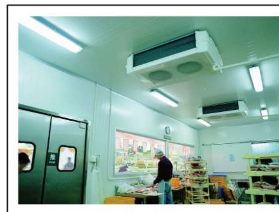
冷藏加工间 Preparation Room
